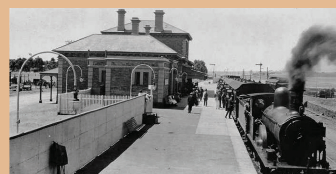
Riverton Railway Station, the site of the tragic shooting event of 1921 State Library of South Australia B68909
